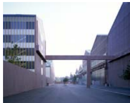
Aqueduct carrying rainwater from the new buildings to storage tanks at the rear of the Lycée © Hélène Binet
