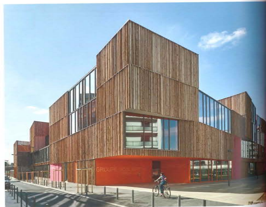
The richly textured façade of the Simone Veil School Complex features rough oak stakes on a grey background, spliced with segments of colour.
