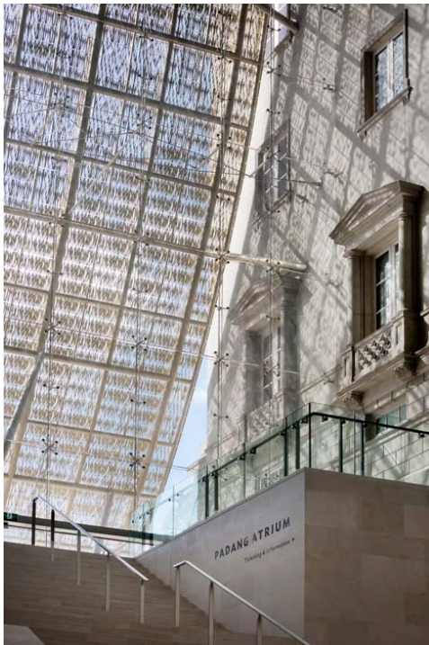
The glass and metalwork continues onto the roof of the gallery and is supported by a series of tree-like structures made from steel.
