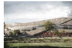
Christchurch Convention Centre Christchurch Woods Bagot, Warren and Mahoney
