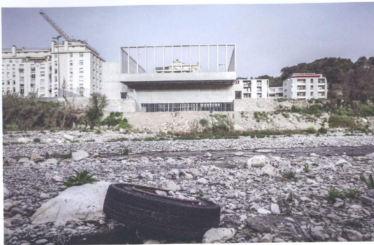
▲ Gymnase Futsal de l'Arianne, Nice, CAB Architectes @ Aldo Ancretti
