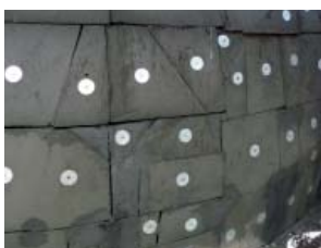
Foamglass et clous provisoire
