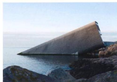
**Sea legs.** In the Norwegian North Sea, some 400 km from Oslo, lies Under, Snøhetta's latest feat, an underwater space housing a 40-seat restaurant and a research centre on marine life. Bolted to a poured concrete base on the seabed, the building is a 34-metre-long monolith, sloping to 20°.
